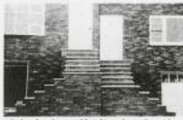
Split level and ground level two house house
